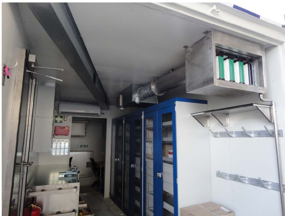
Internal outfitting of the workshop
