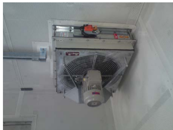
Axial flow exhaust fan capacity 14000 m 3 /hr, with motorized damper
