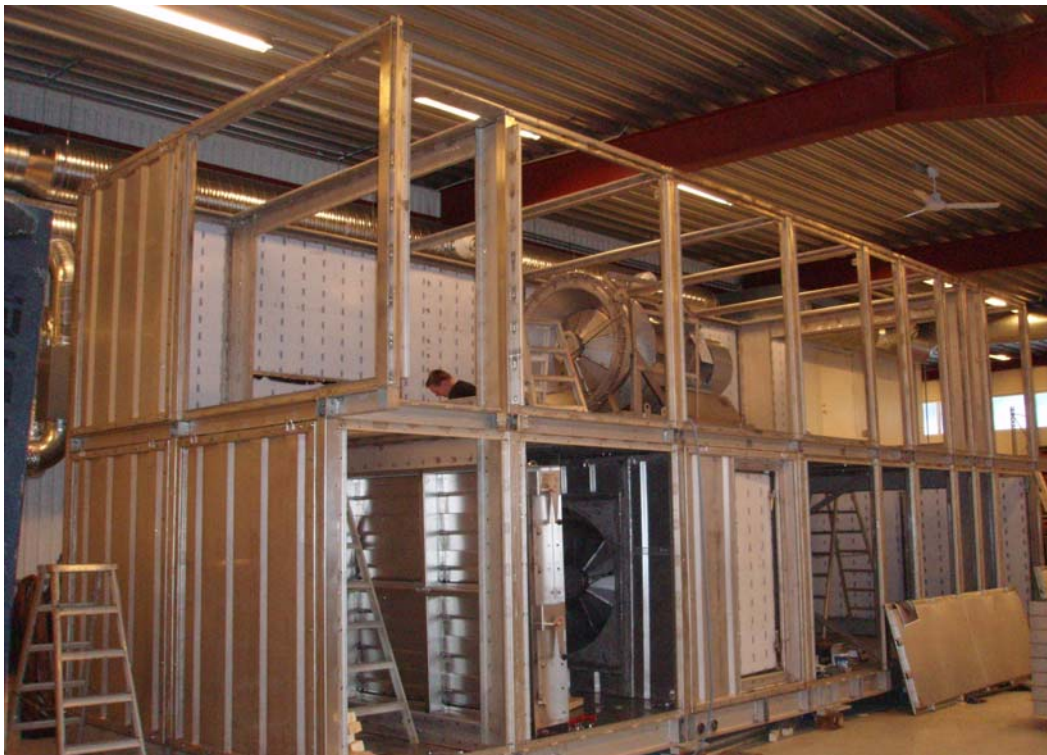
Framework under construction in Trans constructions workshop in Dal
