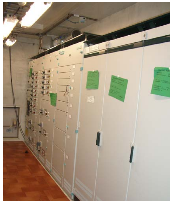
Inside the container, the frequency converters on the left and the 660V switchboard on the right.
