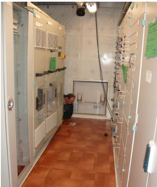
Inside the container, the frequency converters on the left and the 660V switchboard on the right.
