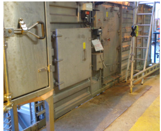
Lower level after installation Offshore, Floor height matching perfectly.
