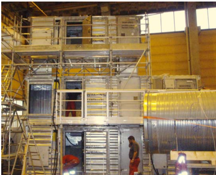
Installation at workshop, nearing completion
