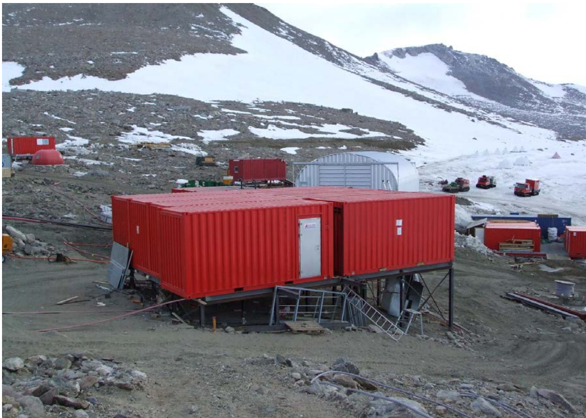
Assembly work nearing completion
