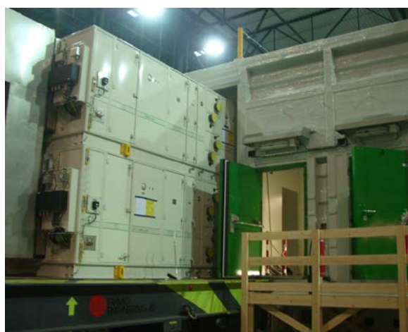
Skidding the Air Handling Units into the module
