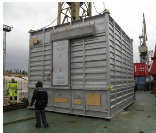
The main entrance was a pneumatic operated sliding door
