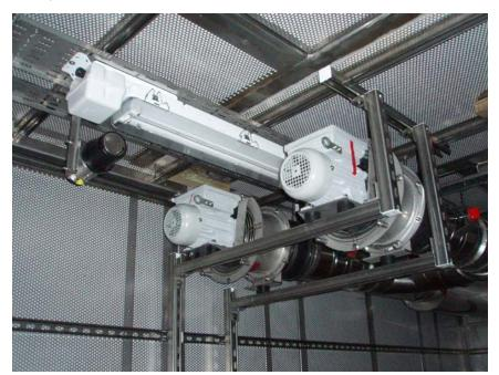
The picture on the left shows the Eexd fans and motors installed on each side of the lighting fixture.
