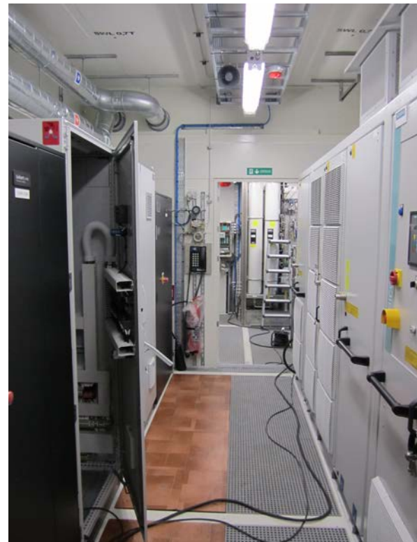
View through the HPU section, false floor clearly visible
