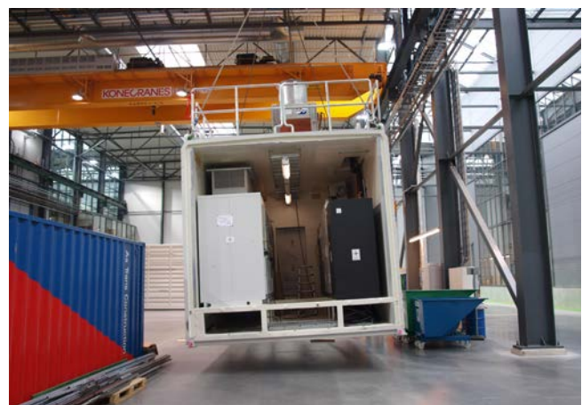
Lifting the VSD section after completion of installion
