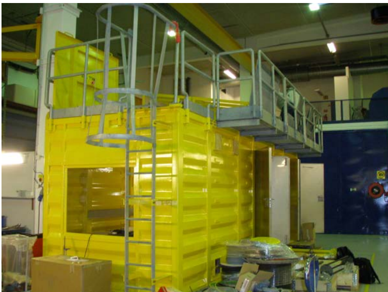
External view showing ladder and walkway on roof.
