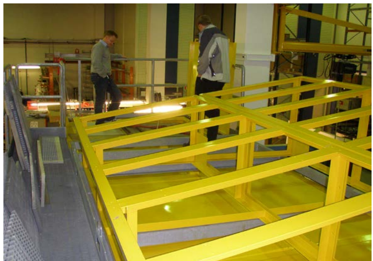
Framework on roof for installation of Solar Panels
