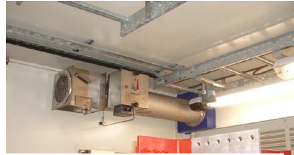
Fresh air supply with fire and constant pressure damper
