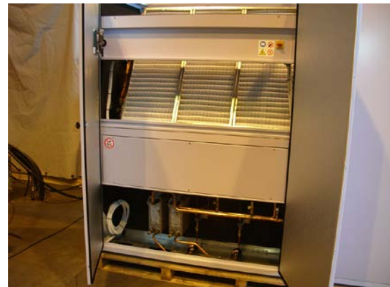
Floor standing 63 kw AC unit ready for installation
