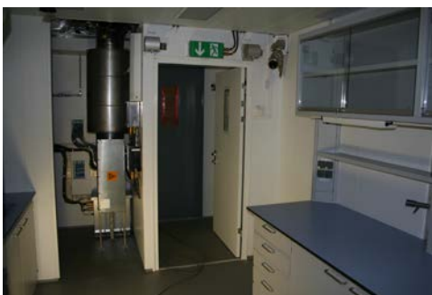
Internal door into air lock
