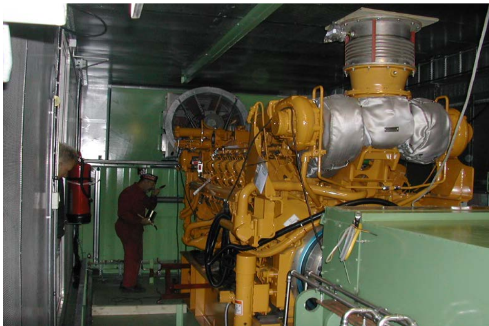
Installation of the generator set, runway beam along the full length of the module
