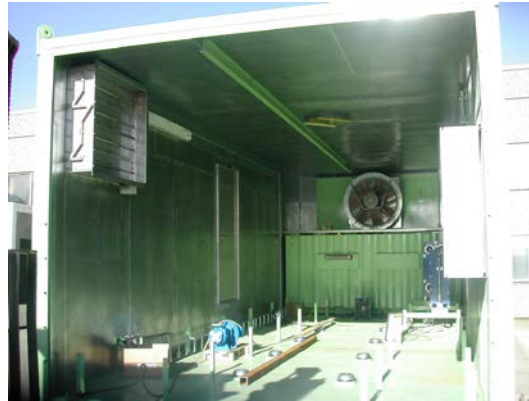
Internal layout prior to installation of generator
