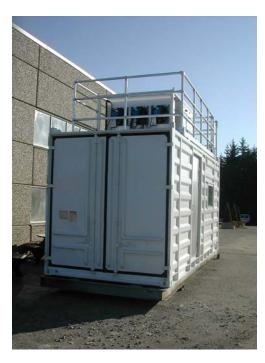
After completion a factory acceptance test is performed using simulated heat generation from the trafo to demonstrate the max internal temperature.
