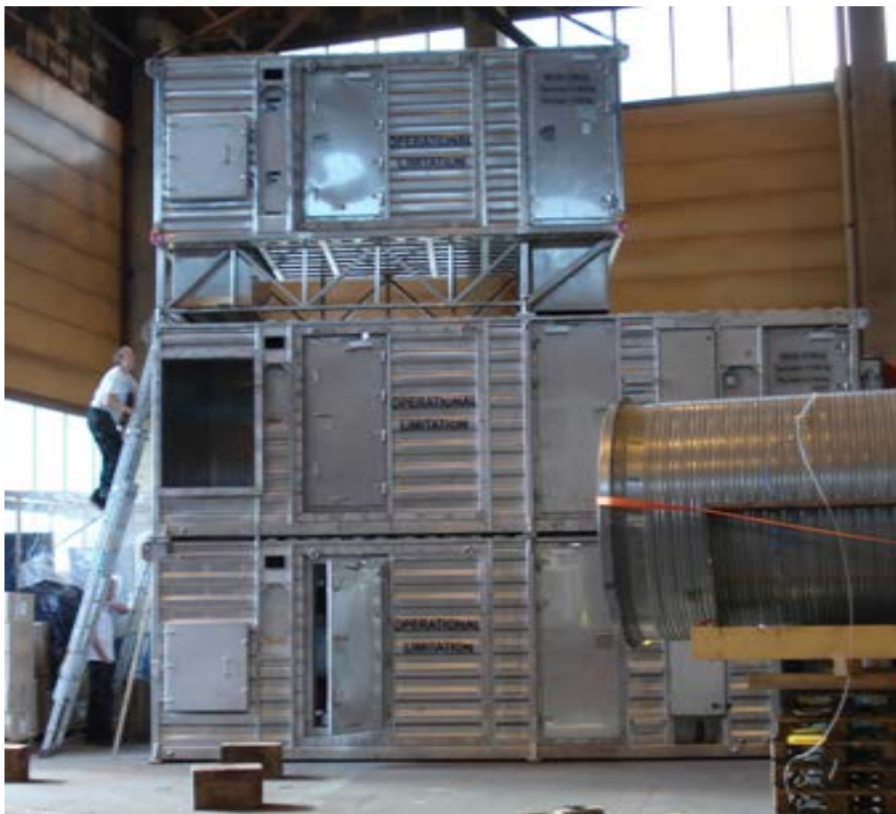
Installation nearing completion
