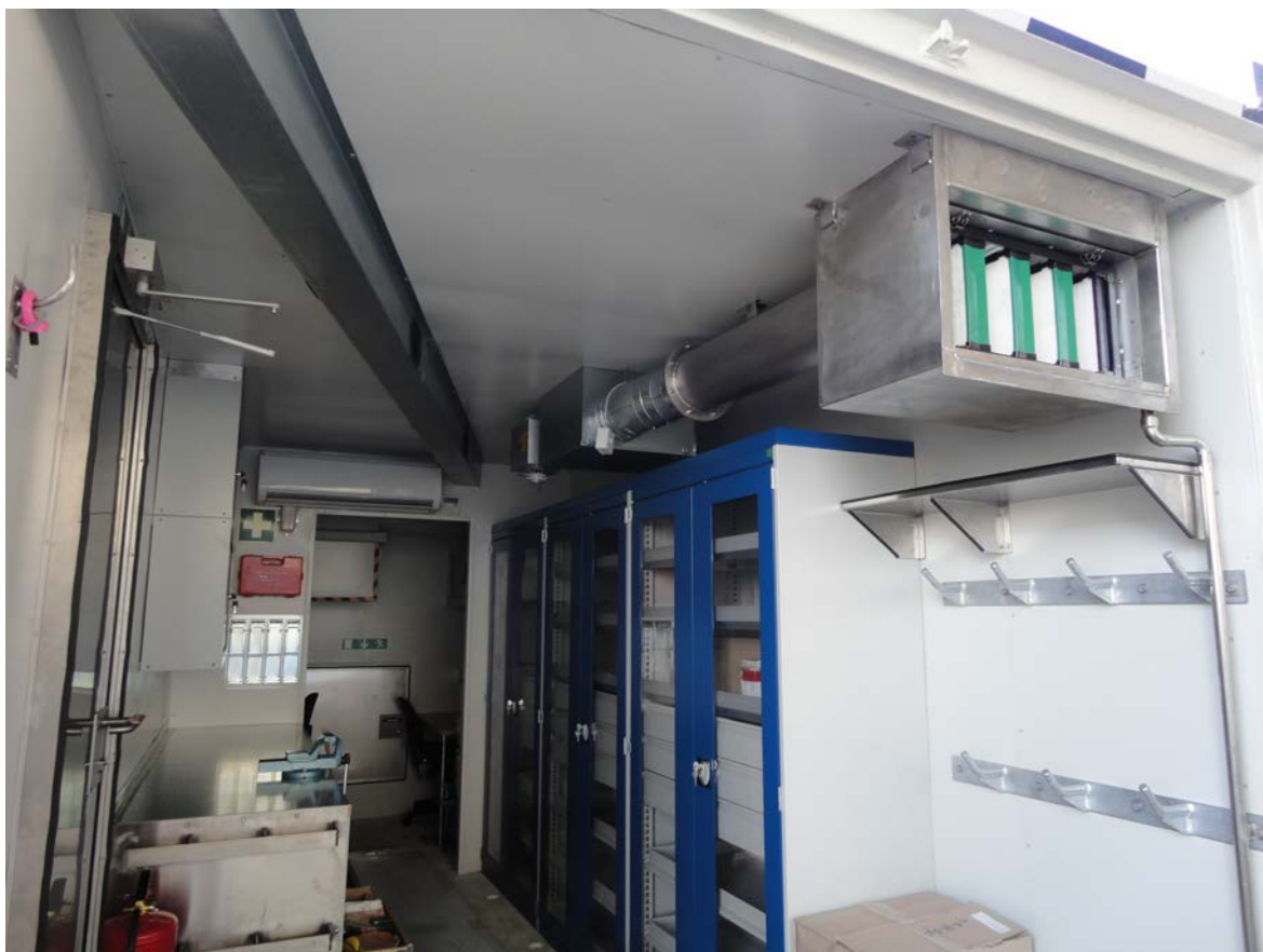
Internal outfitting of the workshop
