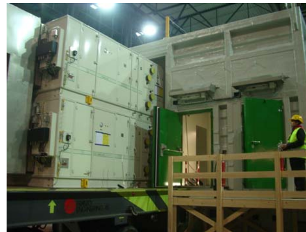
Installation of HVAC Units
