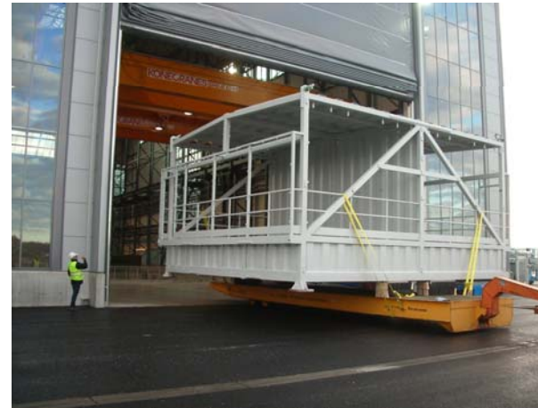
Skidding upper module into workshop
