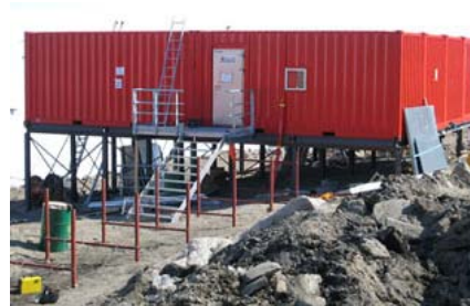
Powerplant, made up of 8 containers, for use at South Pole
